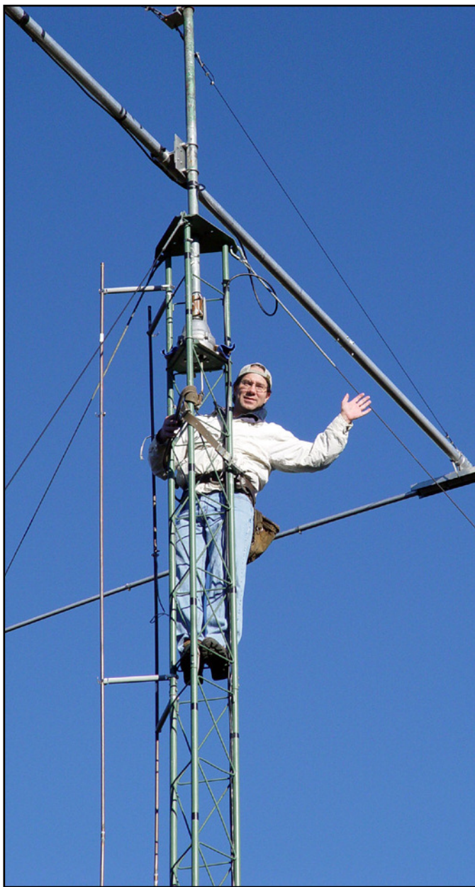
Your author (N0VD) making some adjustments to the 160m shunt feed shorting strap.
