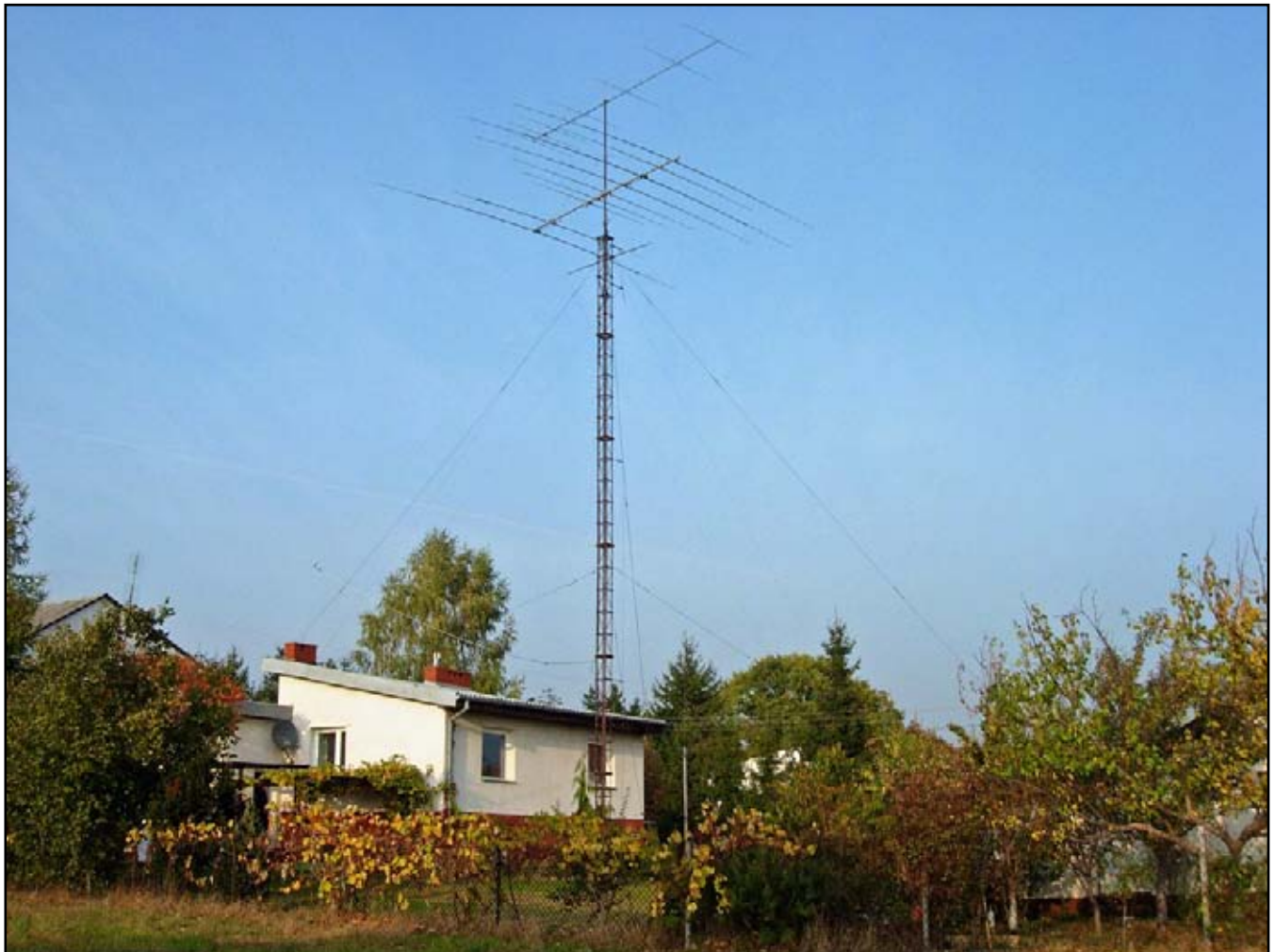
The 160m tower at SP5EWY, in the suburbs of Warsaw. Rys shunt-feeds the tower.
