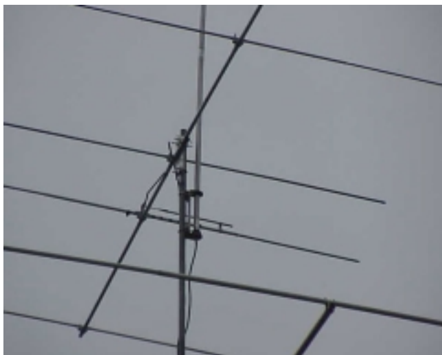
In this view you can see the bracket that supports the 40-meter vertical. It is held on the mast by 2 U-bolts. Loosening these bolts up allowed me to slide the 40-meter vertical up and down the mast. It is about as far up as I can get it now.
