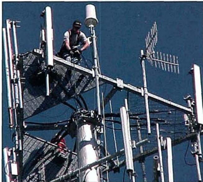
*A SkyExtender installed at the top of a tower. The SkyExtender is the white tube near the tower worker's head. Its relatively compact size, simple interface requirements (Ethernet UTP for power and data), and relatively high power (44.5 dBi) using unlicensed 802.11a spectrum and equipment (with proprietary software and protocols) make it an attractive alternative to Cable and DSL for internet access. (Photo courtesy SkyPilot Network Inc.)*
