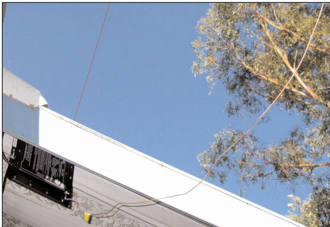
Mounting the SG autotuner at the feed point provides the most efficient tuning and operation. Even though the tuner is weatherproofed, this mounting location under a soffit provides extra protection from direct exposure.
