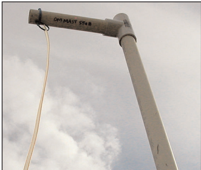
A 6-inch-long piece of PVC extends horizontally from the T-joint at the top of the mast for easy J-pole hanging.
