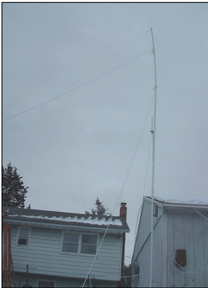
John Mazzone, N2EIK, has had a “35-footer” PVC mast “up for almost a year now” in Kingston, NY.
