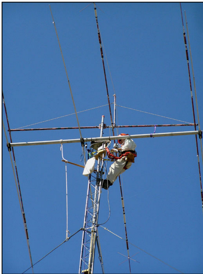
Mike Gross, KØALT's husband, connects a balun to her lowered tribander antenna during a recent tower climbing excursion.
