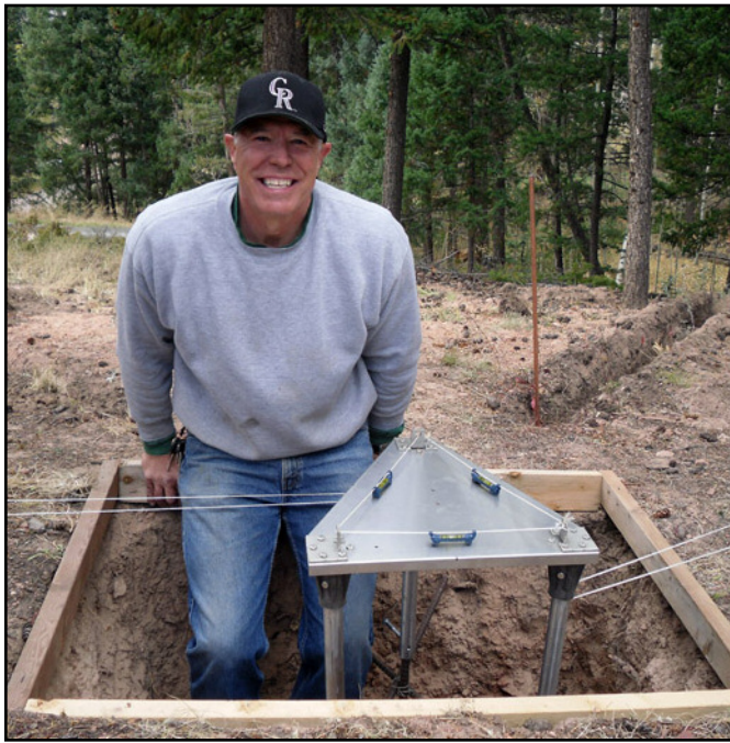
W5JQ leveling the HyTower base.
