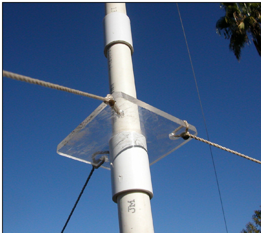
Plastic guy line support points at 6-feet and 12.5-feet along the mast's height help keep the OM's "scoliosis" in check.
