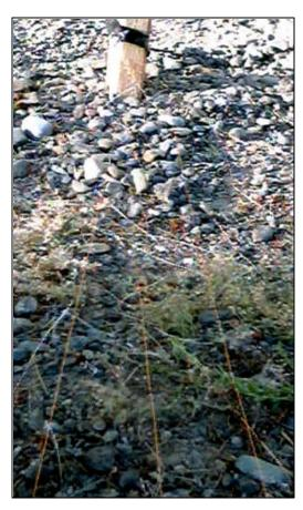
10 wire radials measuring between 40 to 80 feet in length were buried 1 inch under the gravel and then attached/soldered to a 3 inch x 2 inch piece of copper plated circuit board. The board was then connected to the braid side of the coax which was in turn connected to a ground rod, sunk 6 feet in to the earth next to the feed line.
