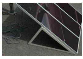
Sed. The mild steel framework is a bit primitive, to say oller the least. It is not adjustable to the proper sun angle, thus you are not going to be able to maximize the amount of sunlight striking the PV array at various latitudes. This mount needs to be re-engineered and made from aluminum to reduce weight.
