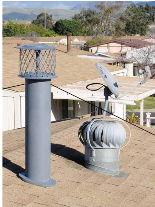
Figure 6a & 6b: 1 Fake fireplace chimney on my roof (see article). It supports part of loop and disguises a VHF/UHF vertical. It looks like it belongs on my roof. The loop wire is emphasized for clarity.
