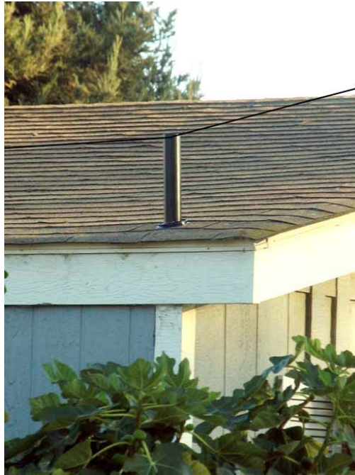
Figure 5: 1 ft. 2 in. ABS DWV plastic pipe standoff glued to a 4 in test cap and attached to the roof with silicone sealant. Neighbors think it's a vent pipe. Loop wire is emphasized for clarity.
