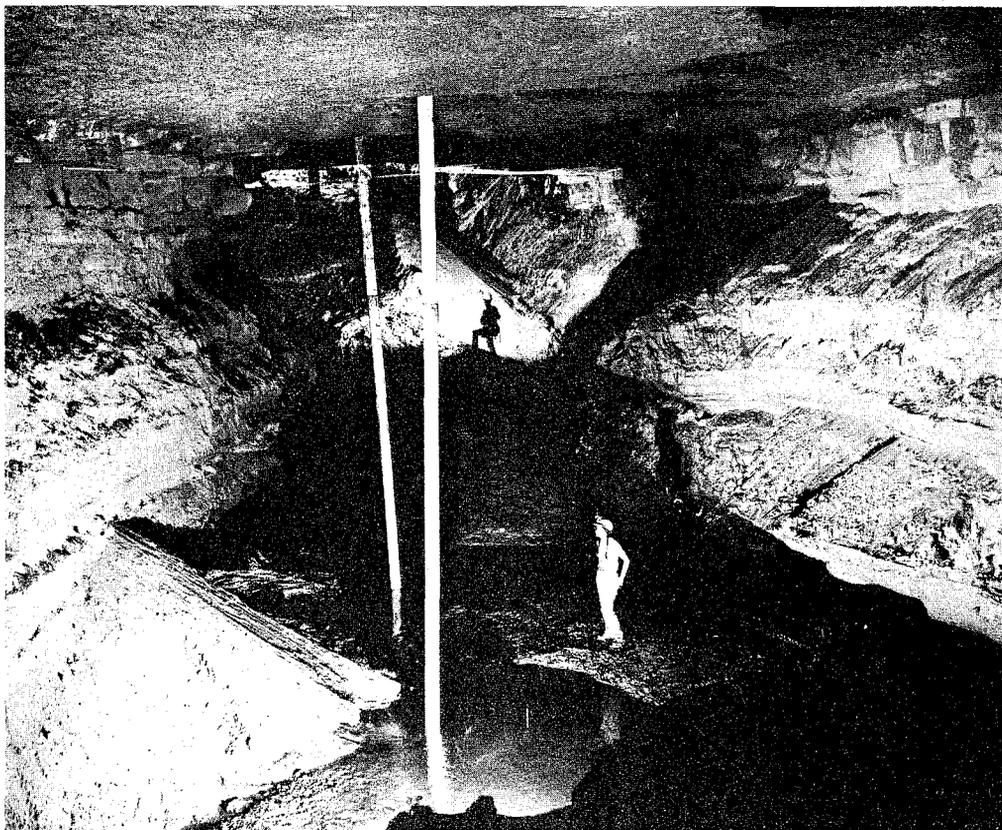
120-foot-deep wells near Park City, Kentucky, penetrated cave within two feet of radio targets. Drill drift caused error. Pipes contain hydrological instrumentation. (Photo by Samuel S. Frushour)
