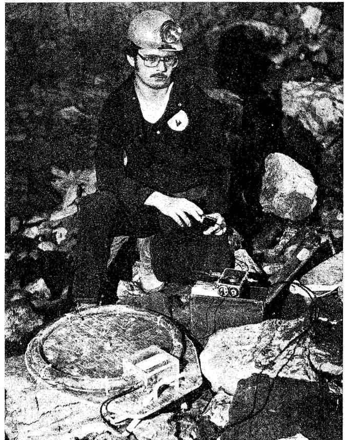
WB9TLH operates underground transmitter on 3500-Hz CW, using microswitch for telegraph key.
